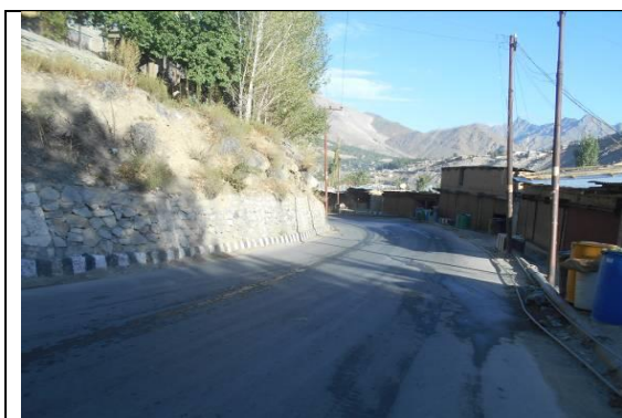
Built-up at Km 1.200
