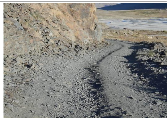
Hilly Terrain at Km 203+100
