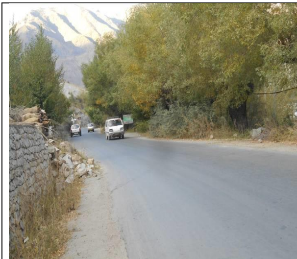
Fair Condition of Road at Km 1+800
