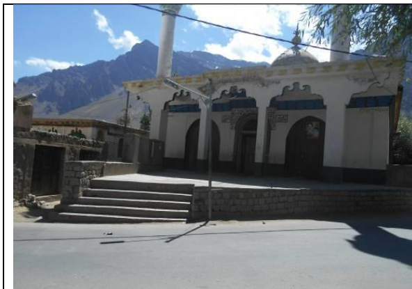
Mosque LHS at Km 19+253
