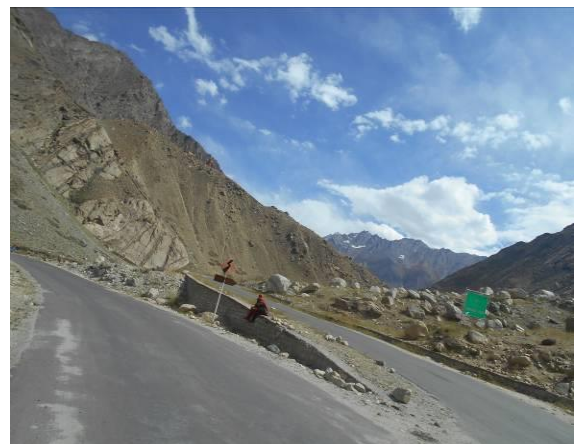
Junction at Ch. 41+915
